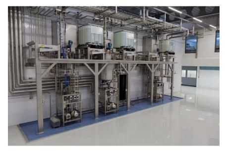
Figure 5: Process vessels and stacked raw material containers at 1st floor level in not classified basic hygiene zone as back side of Figure 5.
