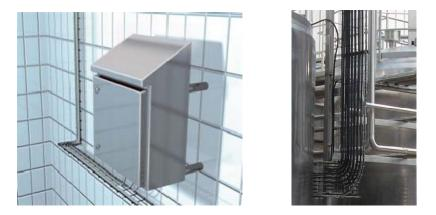
Figure 2: Cleanable arrangements of control cabinet and cabling
