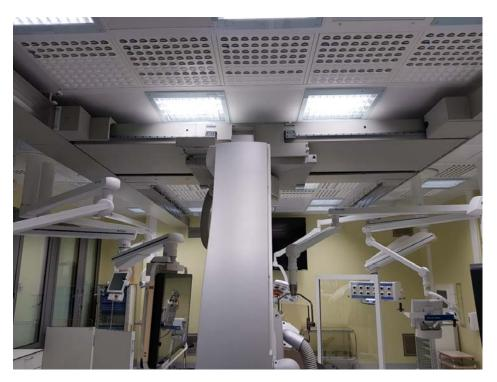
Figure 1 Hybrid Operating Room in Nya Karolinska Hospital, Stockhom, Sweden, equipped with Halton Vita OR Space 5 ventilation system
